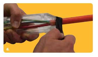
Use the supplied tape to seal the ends of the shell.
