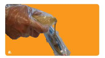
Pour the RAPID 4300 or RAPID 6000 into the shell until it is filled.
